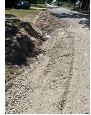
CR 2454 -Before and after the new culvert was installed.
