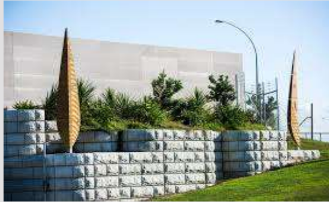
Decorative Retaining Walls
