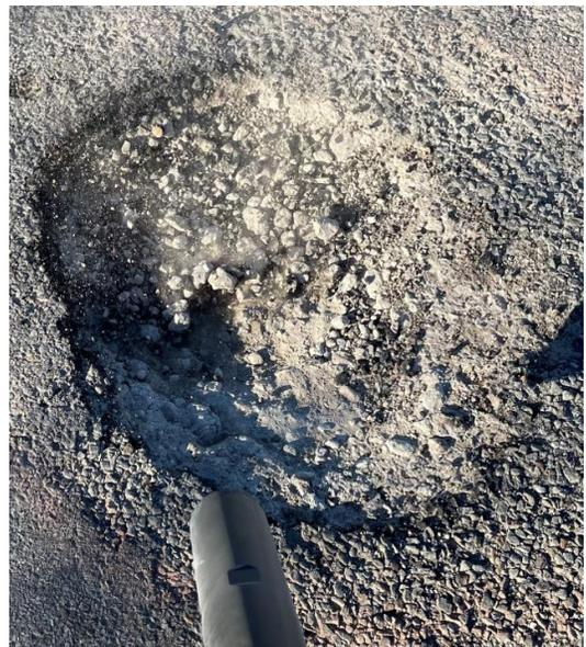
Step 3, Open a bucket of Asphalt Bonding Agent called "Tack" (HomeDepot.com Asphalt Bonding Agent SS-1H Tack Coat (\$50.92 each) and using an old stiff bristle broom, dip that broom into the "tack" and thoroughly "paint" the inside of the hole. Make sure that you cover the upper sides of the hole and even over the top of the pothole.
