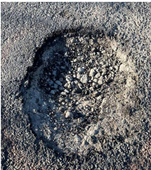
Step 2, use a gas or electric blower to blow out all the loose material from inside the hole
